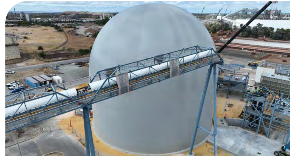
New clinker import circuit under construction at KBT
