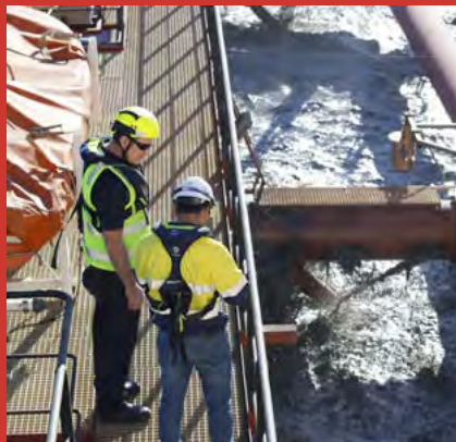
Port Hydrographer Jay Illingworth and Deputy Harbour Master Suraj Joshi supervise the dredging
