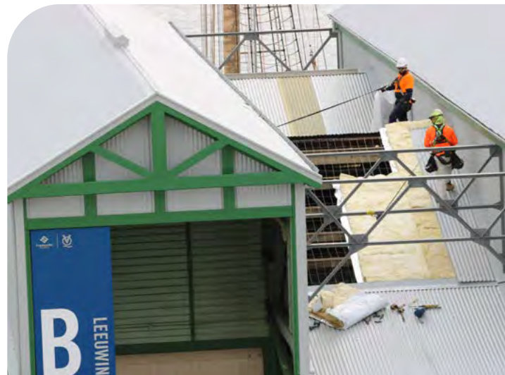
B Shed remediation began in 2023
