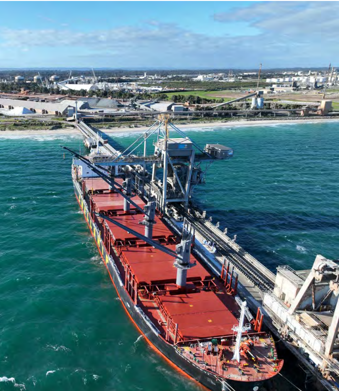
Bulk carrier alongside at Kwinana Bulk Terminal.
