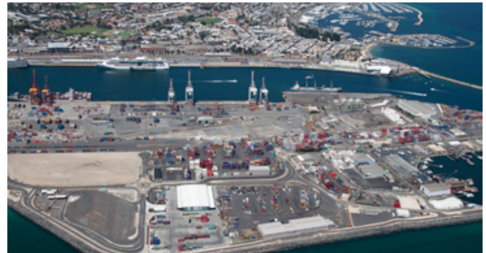
The development of sites on land reclaimed at Rous Head is close to completion.
