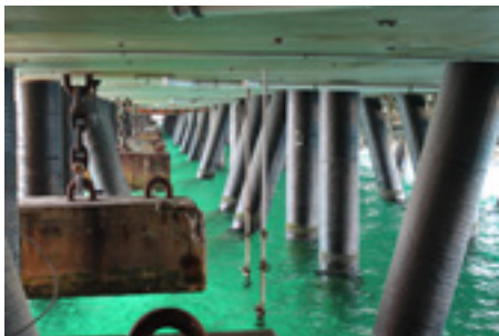
Gravity fenders at the Kwinana Bulk Terminal have been repaired.
